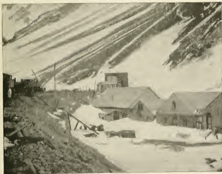
ENTRANCE TO ANDINE TUNNEL, CHILIAN SIDE
